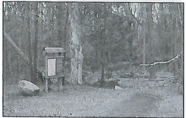
Renovated entrance with tree damage from storm, Sandy
